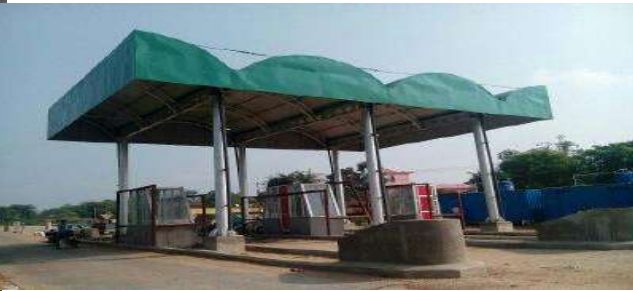
← OVER HEAD GANTRY
